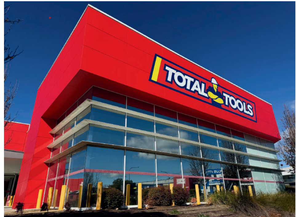
Total Tools - Full Retail Exterior Repaint
