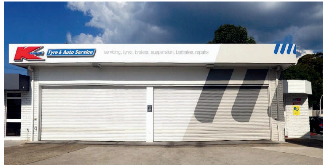
Kmart Auto Commercial Exterior Repaint
