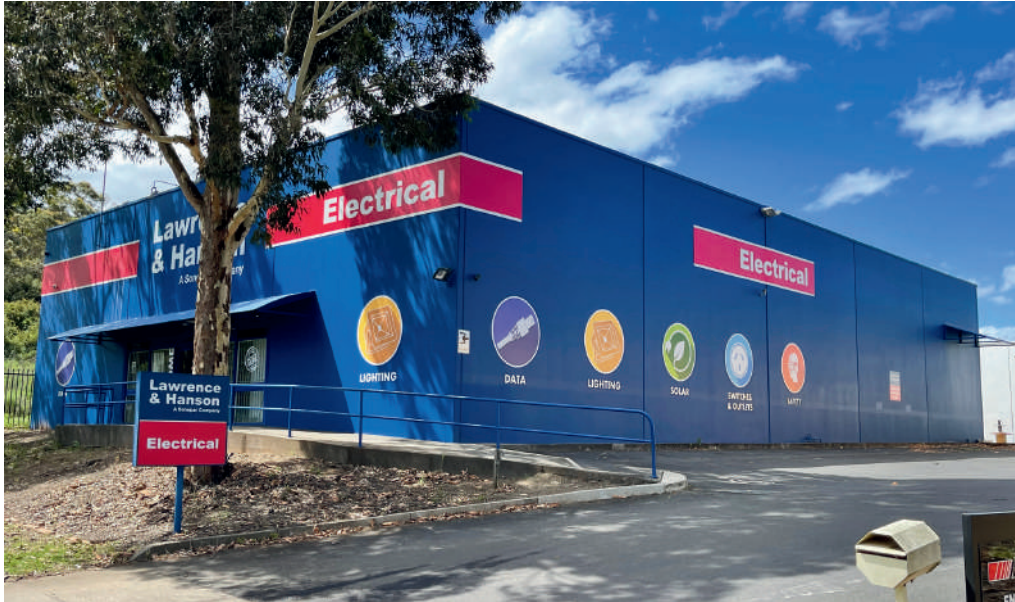
L&H Electrical - Commercial Full Repaint
