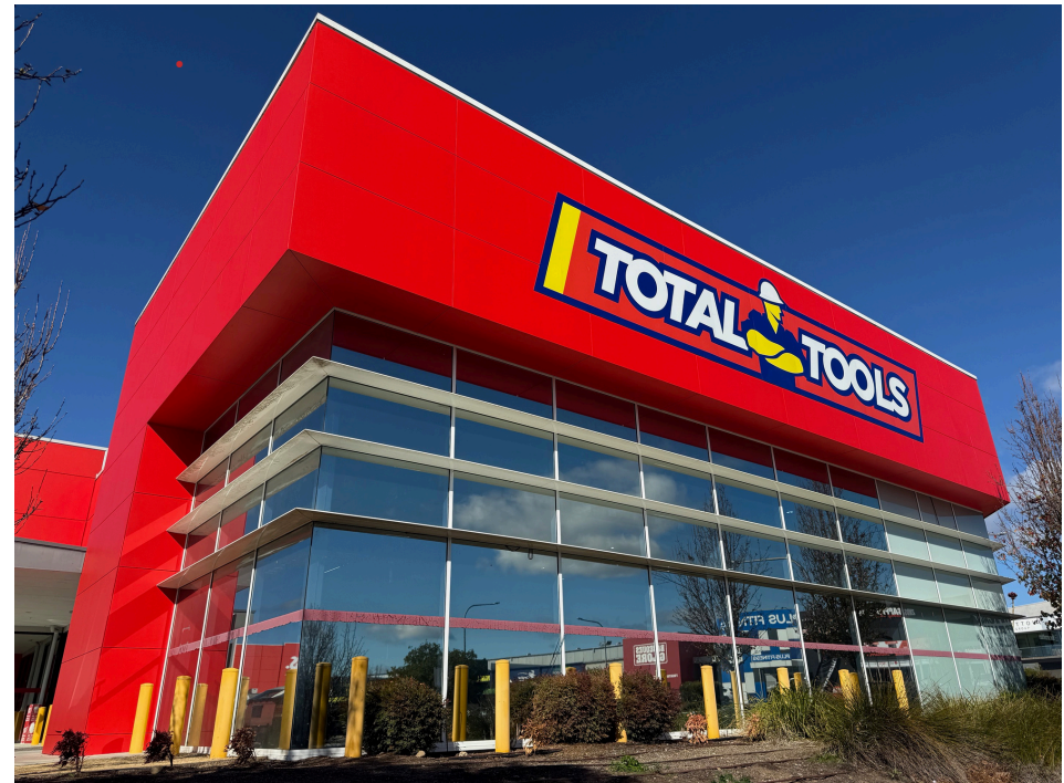
Total Tools - Full Retail Exterior Repaint
