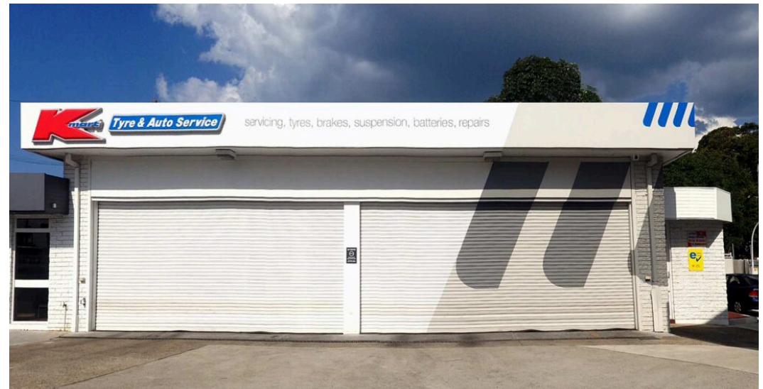
Kmart Auto Commercial Exterior Repaint
