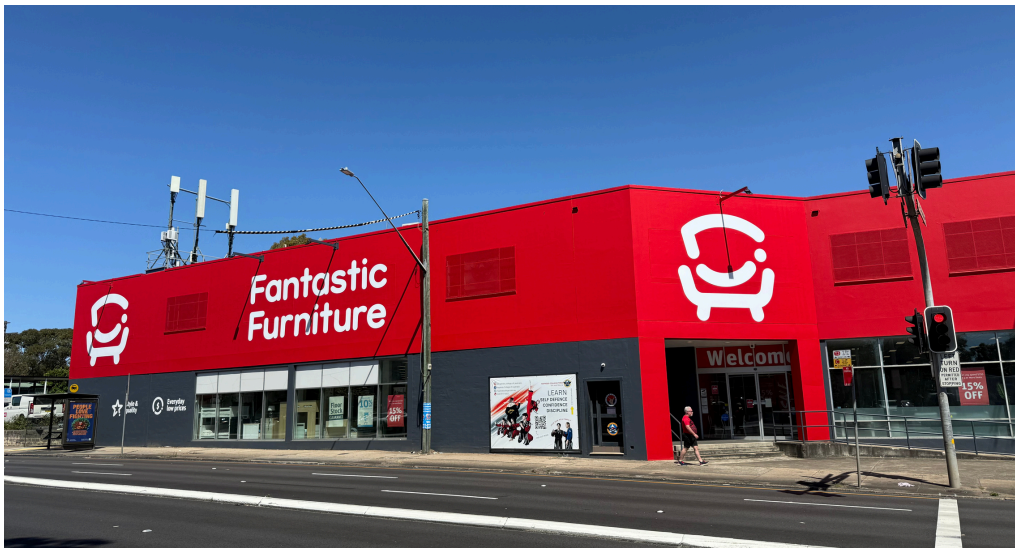
Fantastic Furniture Commercial façade Repaint
